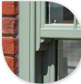
Run through sash horns
